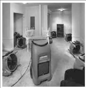
Structural Drying
